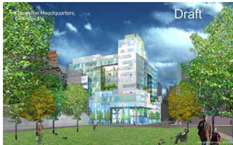
Figure 22: The Genzyme Headquarters in Boston, Massachusetts, was analyzed for cladding pressures when selected critical windows were assumed open during a design storm.
