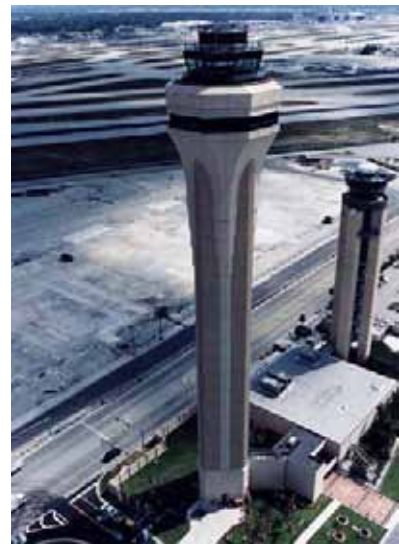
Figure 11: New Miami Air Traffic Control Tower with the old tower in the background.
