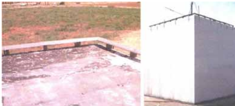
Figure 16: Spoiler on the edge of the TTU Building in Lubbock, Texas (after Banks Sarkar Wu and Meroney, 2001).
